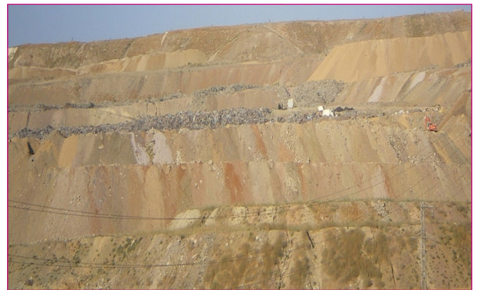
Photo of covered Mamak landfill site after rubble is arranged into dams (Source: ITC)
